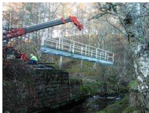
The new bridge over the Altyre Burn
