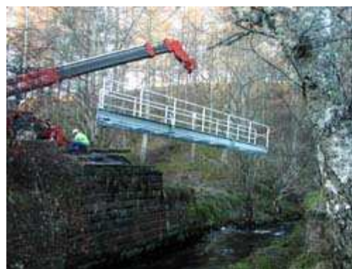
The new bridge over the Altyre Burn
