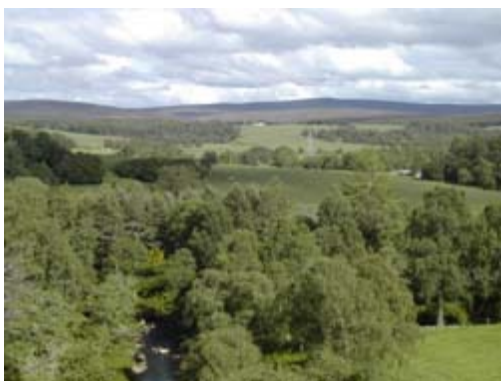
River Divie looking east from the Divie viaduct
